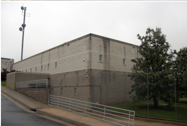
Side – before and after
